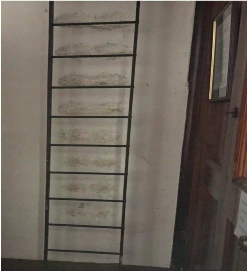
Figure 11: Steel Ladder Up to Bell Tower
